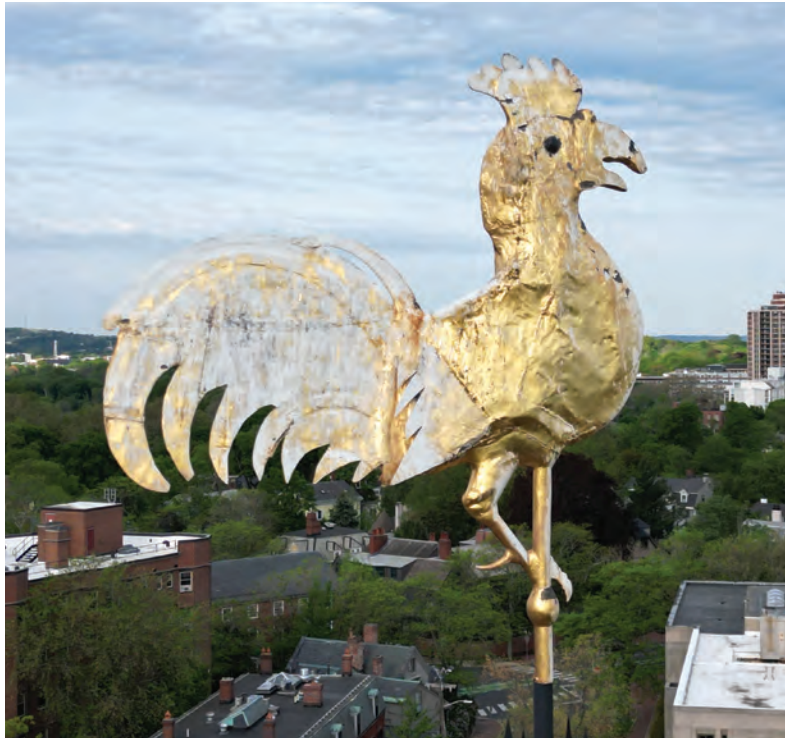
A drone image made on May 1, 2023, showed significant erosion of the gilding, especially to the tail feathers, on this side of the cockerel weathervane.
